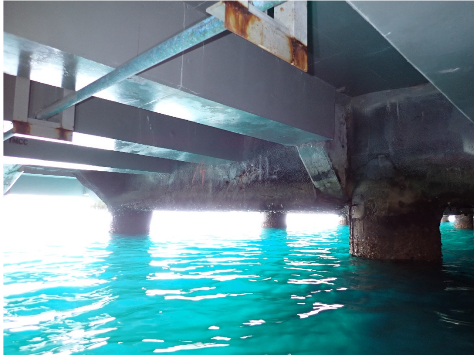
Photo 1: Typical Pier Substructure at Pier 10
